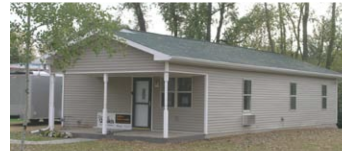
This Habitat and Thrivent Builds home was built in Shawano in 2007. We’ll soon be starting a new Thrivent Builds home in the Village of Tigerton.
